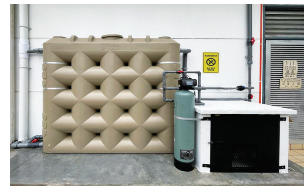
Rainwater harvesting system installed at PETRONAS station
